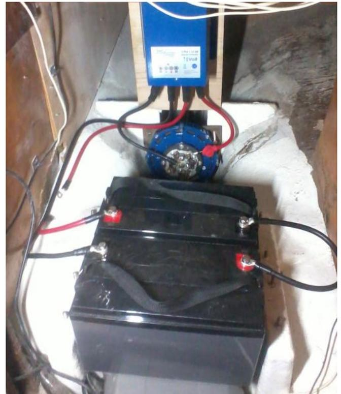
**Controller, motor and battery bank**
